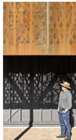
Detail that nods to qualities of the original features of the building. The old latticework has been re-imagined in annealed steel.
