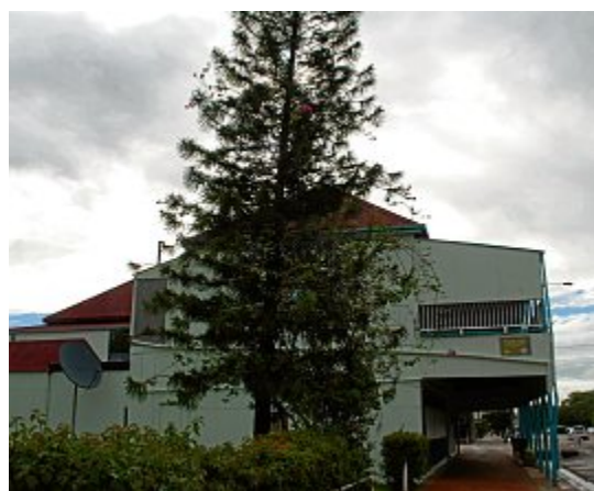
2010: After last drinks, The Globe faced demolition. An unsuccessful attempt was made to gain Heritage status for the historic pub, but in the end, it was rescued by a sensitive re-development concept.
