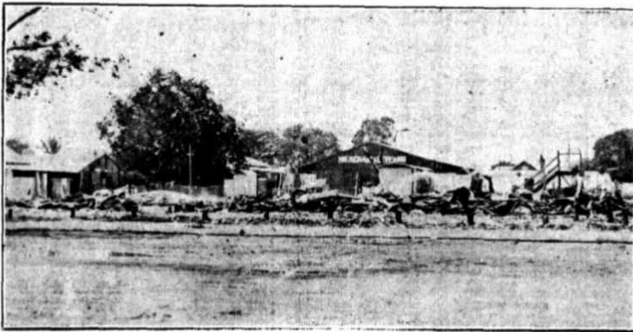
Front View showing the charred stumps of verandah posts..
